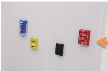
Pull handle for manual actuation of fire alarm
