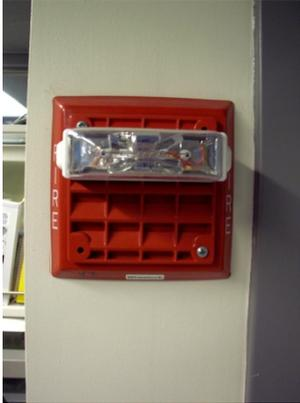
Figure 4: White strobes for fire alarm system
