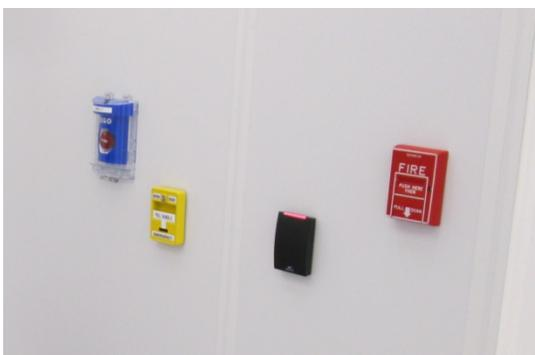
Figure 6: (From left to right) Emergency gas off station (blue), emergency door unlock (yellow), and fire pull station (red).
