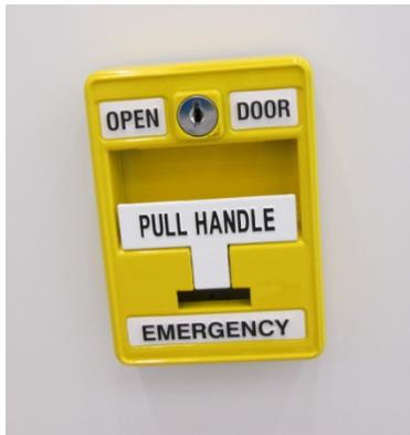
Figure 14: Pull handle to unlock emergency exit doors
