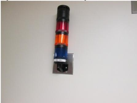
Figure 5: Light tower for gas alarm system
